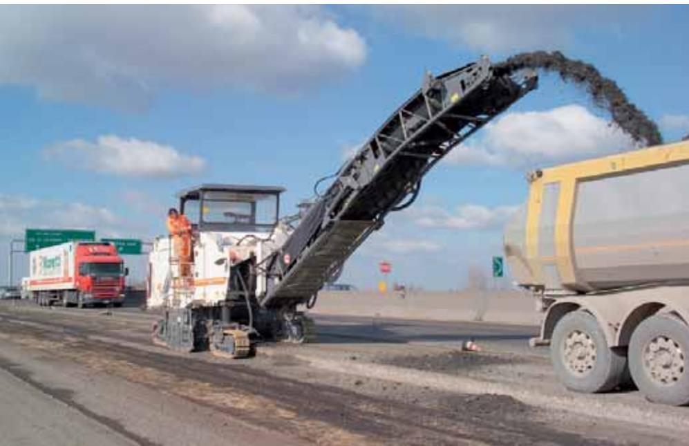
Figure 6 – Road milling machine.
